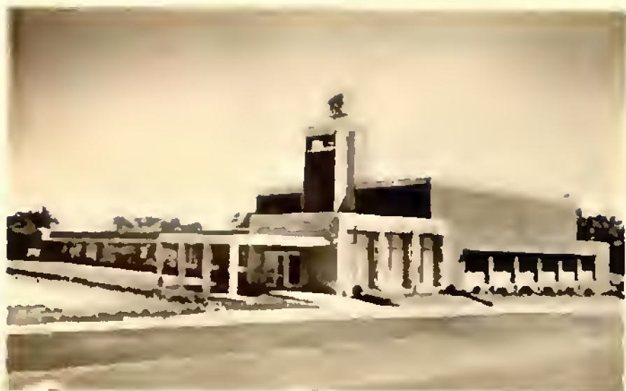
New WDBJ-TV Studios, among the largest and most modern in the entire South. Finest technical equipment — 316,000 walls e. r. p. — CBS affiliate.
